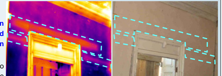
FRONT DOOR - HOTTER (LIGHTER) RESPONSES HIGHLIGHTING THE POSITION OF THE INTERIOR DOOR LINTEL, AND ALSO TIMBER INSERTS BELOW
